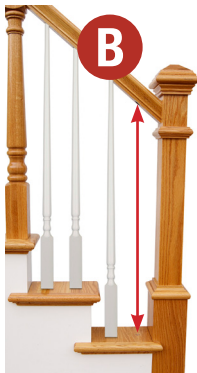
Remove old wood baluster. Measure and cut new metal baluster.
